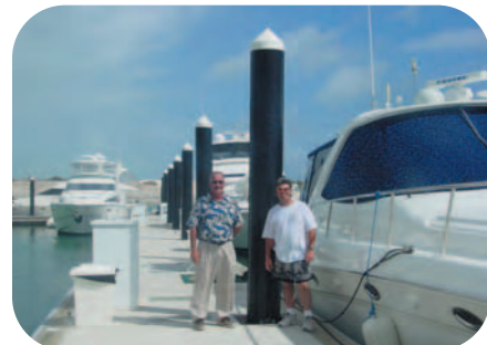
Bob Yeager, Emerald Bay's Director of Construction, left, with Randall Chapman, President of Fluoron after inspection of a row of UHMW-PE covered pilings.
